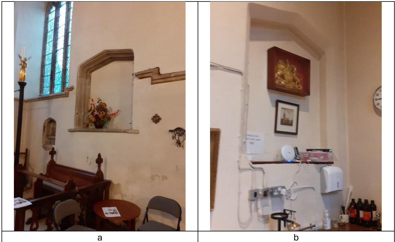
Figure 2. The blocked up window structure. a – from the Lady chapel; b – from the vestry. The bottom edge is at the same level in each case.
