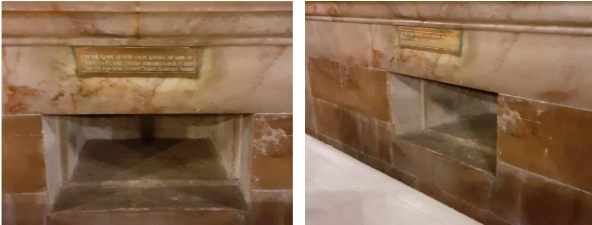
Figure 1. The slot in the wall at the east end marking the position of the “cupboard”
