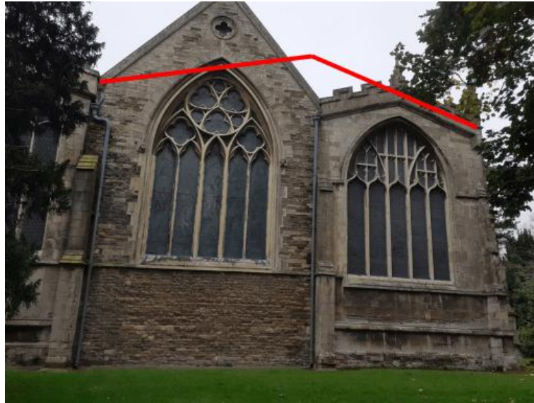
Figure 5. Photograph of the east end of the church showing the roof line of the 1851 model.
