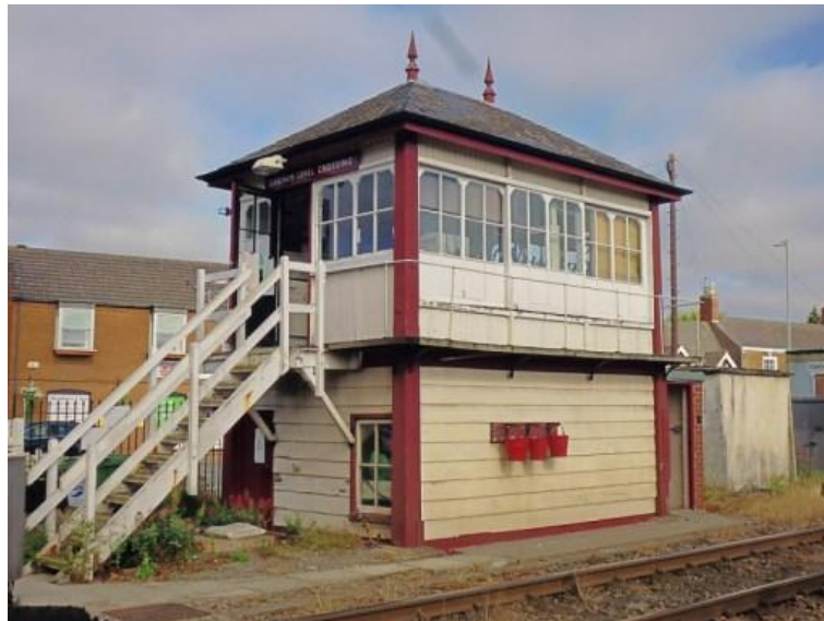
Figure 6. Oakham signal box at the site of the Northgate Cross
