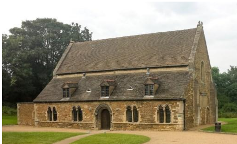
Figure 4. The Great Hall of the Castle from the south
