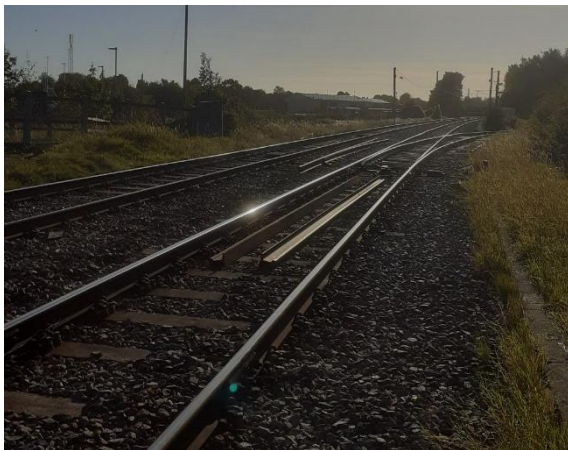
Looking south from the Burton Old Road crossing
