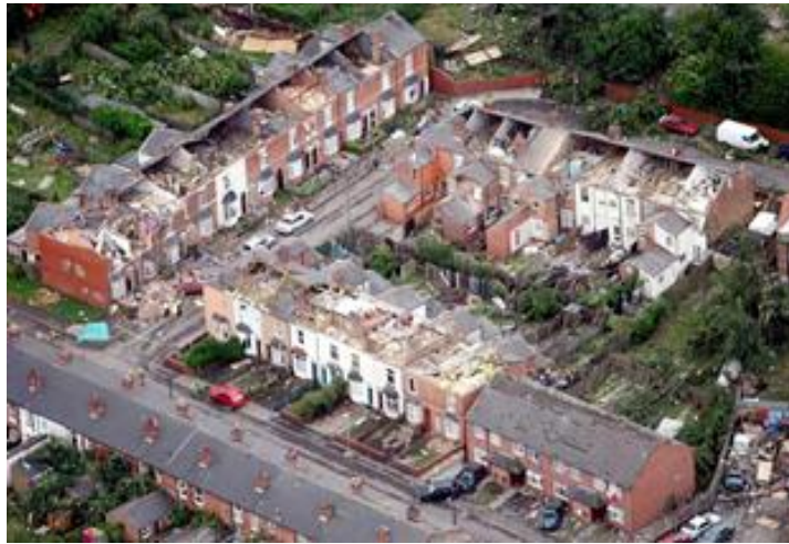
Damage caused by the Birmingham Tornado
