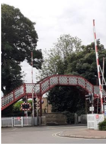
A. The railway crossing
