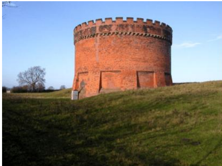
Figure 7 Kilsby tunnel airshaft
