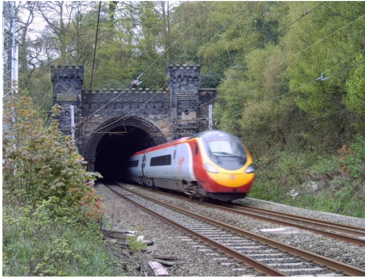
Figure 6 Western portal of Shugborough tunnel
